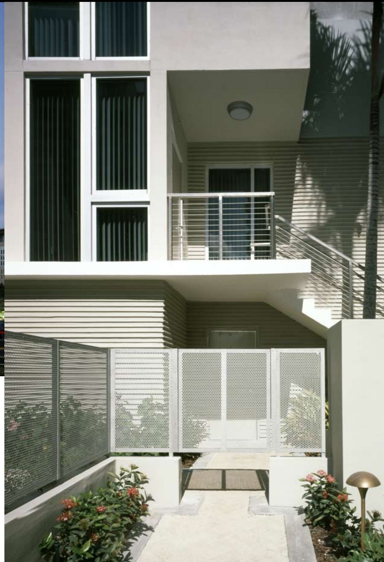
(LEFT PAGE) View from south east (RIGHT PAGE) View of unit entry from West Avenue
