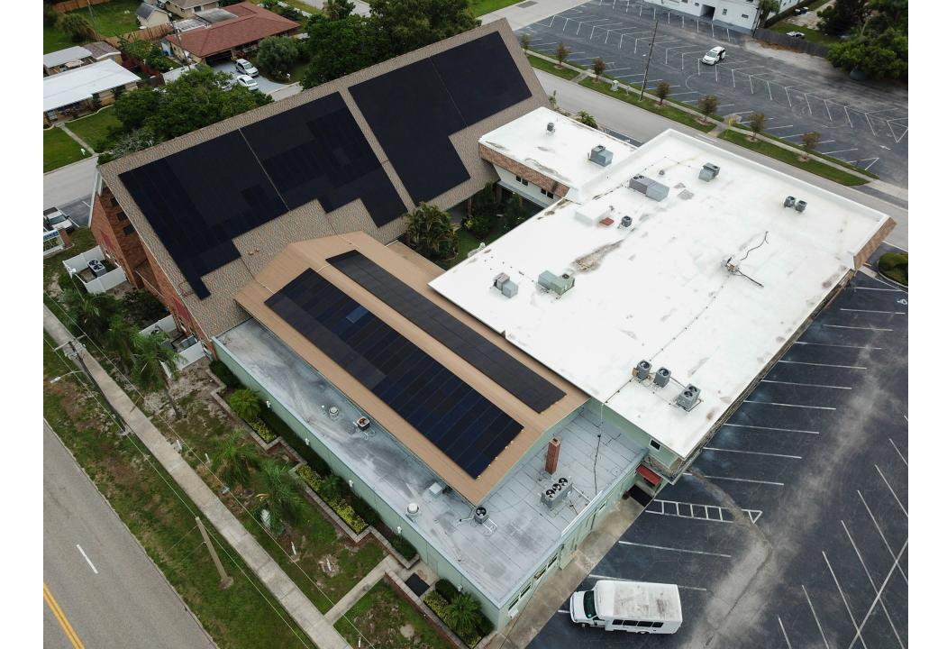
System 391 x Hanwha 340 Solar Modules with Enphase Microinverters.
