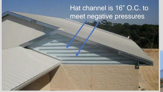
Note the additional framing for the soffit panels
