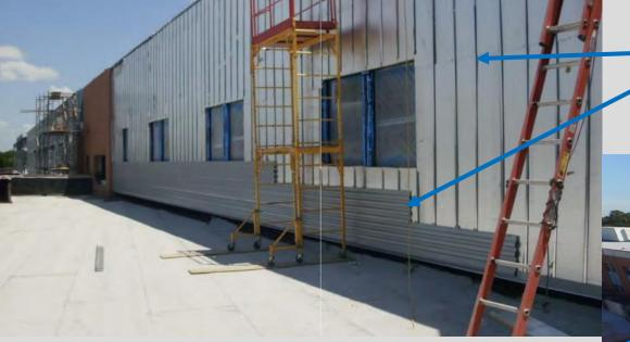
Pre-determined flashing breaks incorporated into design
