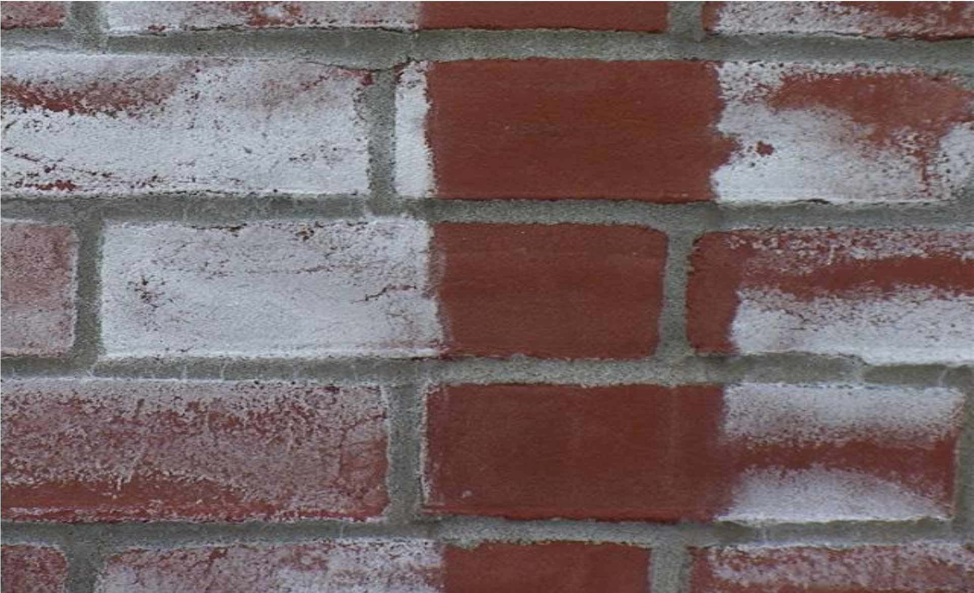
Efflorescence
