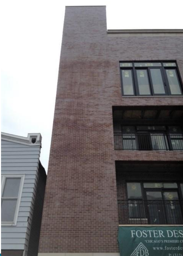
Iron Spot improperly cleaning restored with OneRestore
