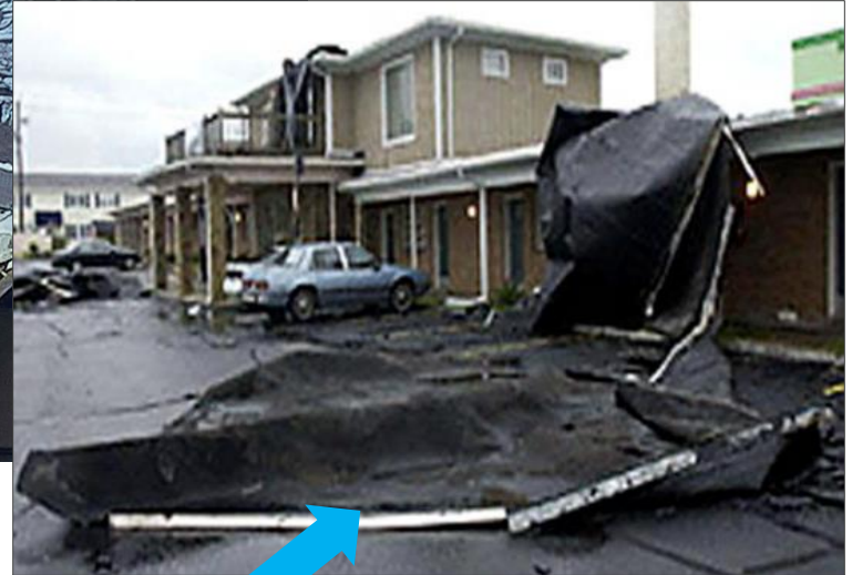
Gutter Pulled Free
