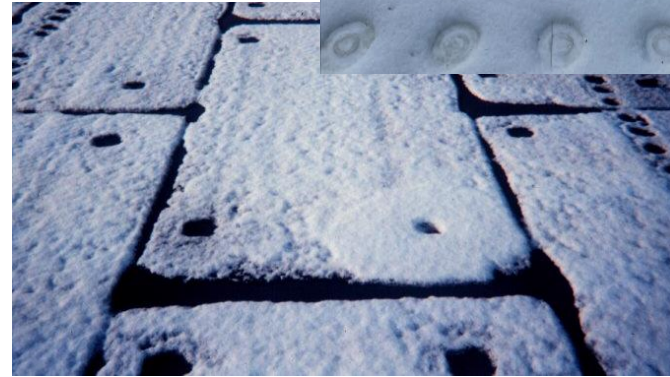
Thermal Loss of rigid insulation which has been mechanically fastened.
