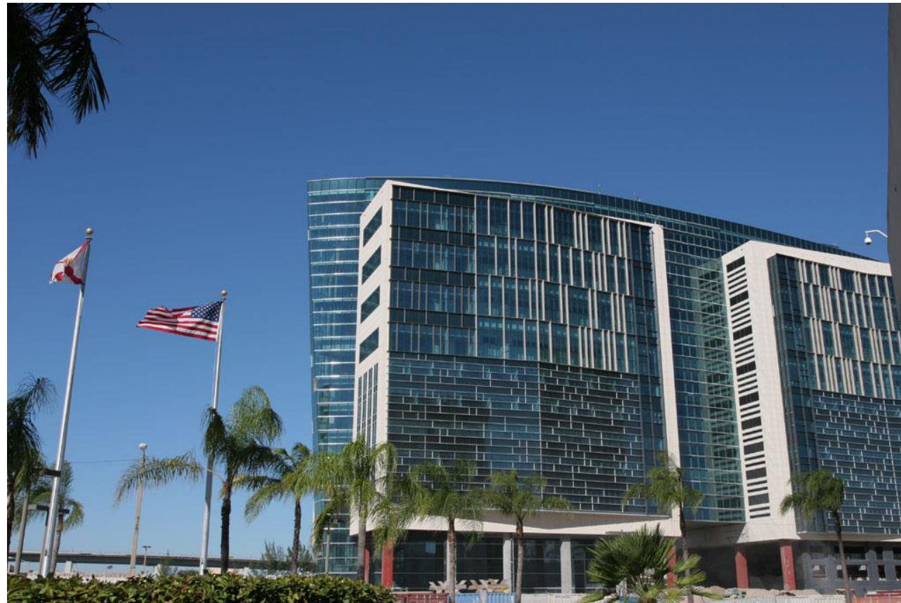
Wilkie D. Ferguson Federal Courthouse Miami, FL
