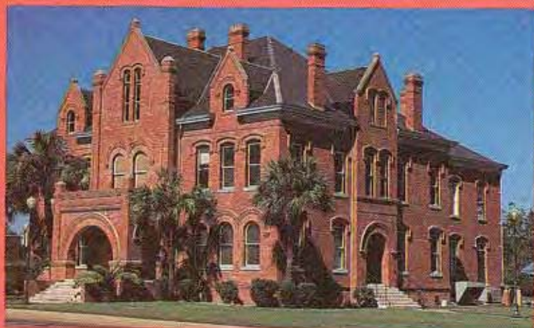
Old Calhoun County Courthouse ♦ Frank Lockwood and Benjamin Bosworth, architects 1904, Blountstown With its solid massing and arches, the Romanesque Revival style was particularly popular for civic buildings.
