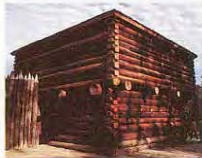
Fort Foster ← Originally built 1836, Vicinity of Zephyrhills
