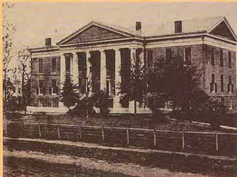
◆ Florida's Capitol Cary Butt, architect 1845, Tallahassee
