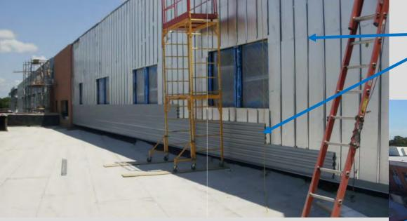
Pre-determined flashing breaks incorporated into design
