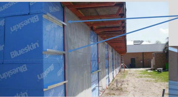
Adequate attachment spacing because wind load requirements determined up front by structural engineer
