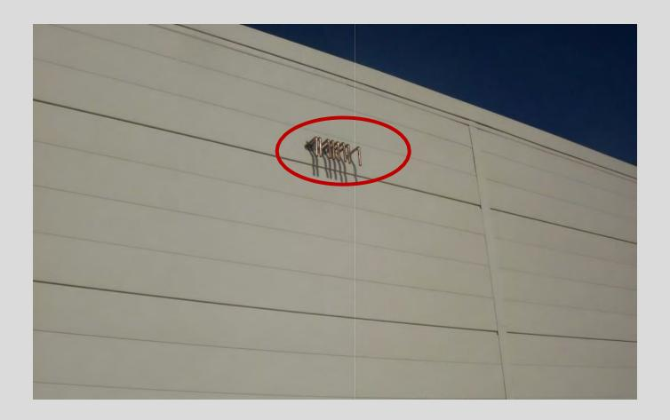
Extensive flashing detail design, followed by poorly executed penetration details
