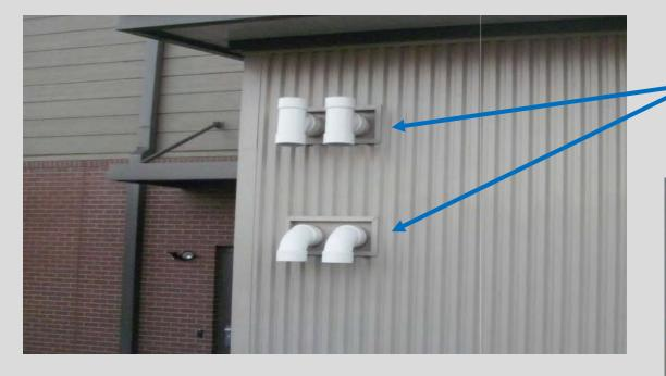
Clean, neat and weathertight flashing details on penetrations
