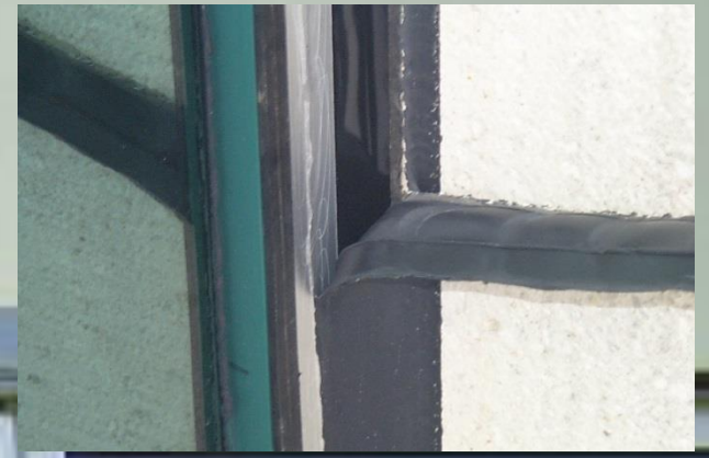
WEATHER SEAL DEGRADATION
