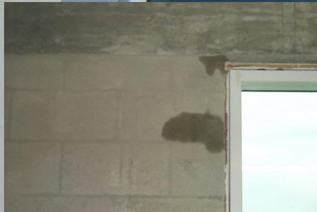
LEAKS DUE TO POOR SYSTEM DESIGN
