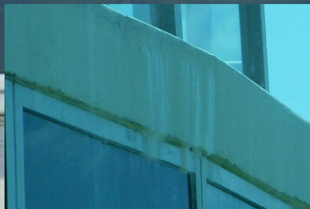
LEAKS DUE TO SURROUNDING CONDITIONS
